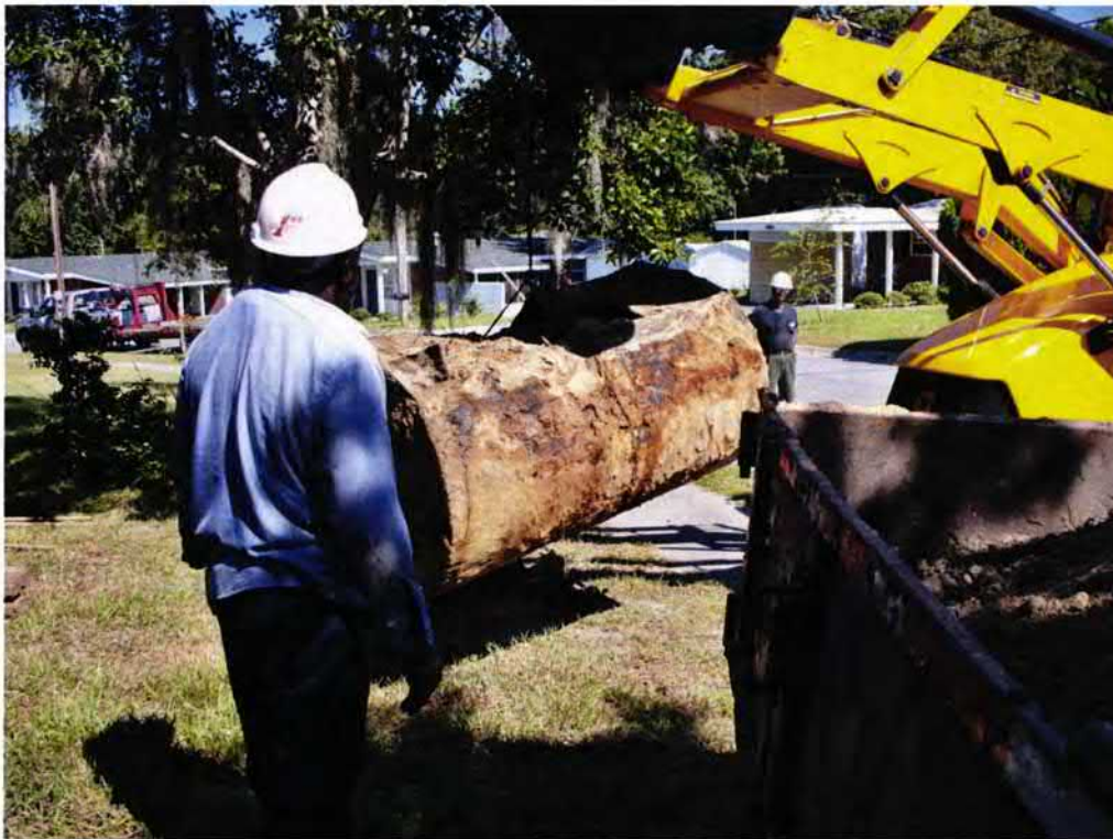
Picture 2: UST 742Bluebell.
